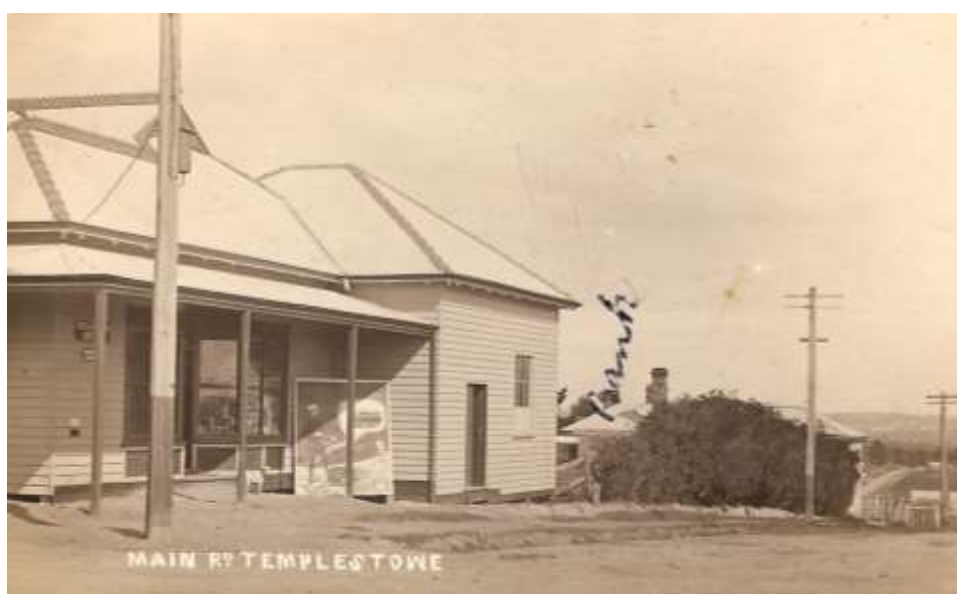
Figure 3: South-west corner James and Anderson Sts, Templestowe, showing General Store, Laver's Bakery and Templestowe Hotel behind far right pole
