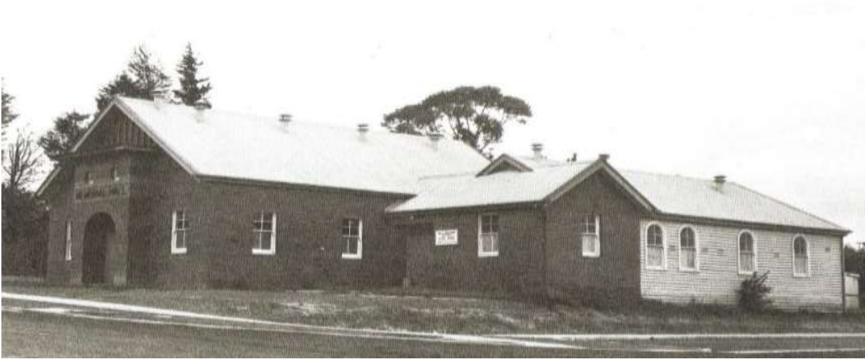
Figure 5 : Templestowe Memorial Hall
