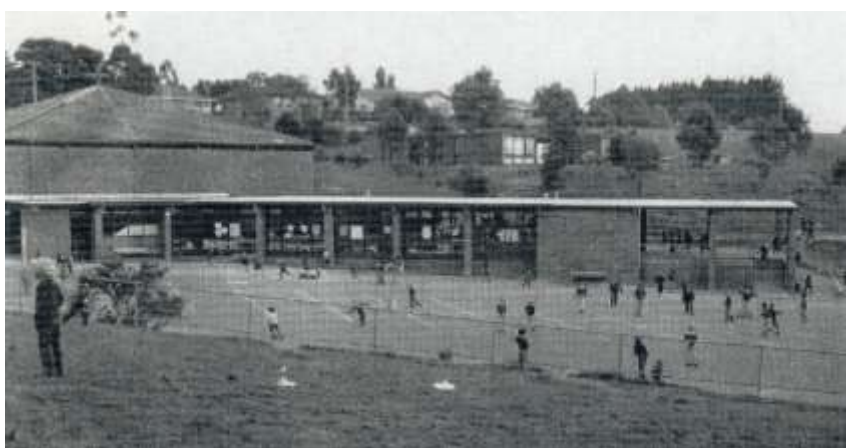
Figure 46: School yard, showing 1977 Junior School Extensions
